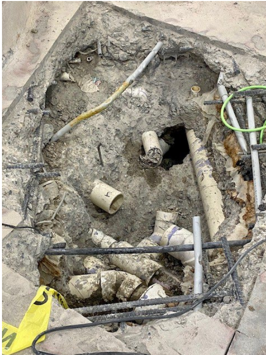
Image 1 (before repairs, broken pipes removed)
